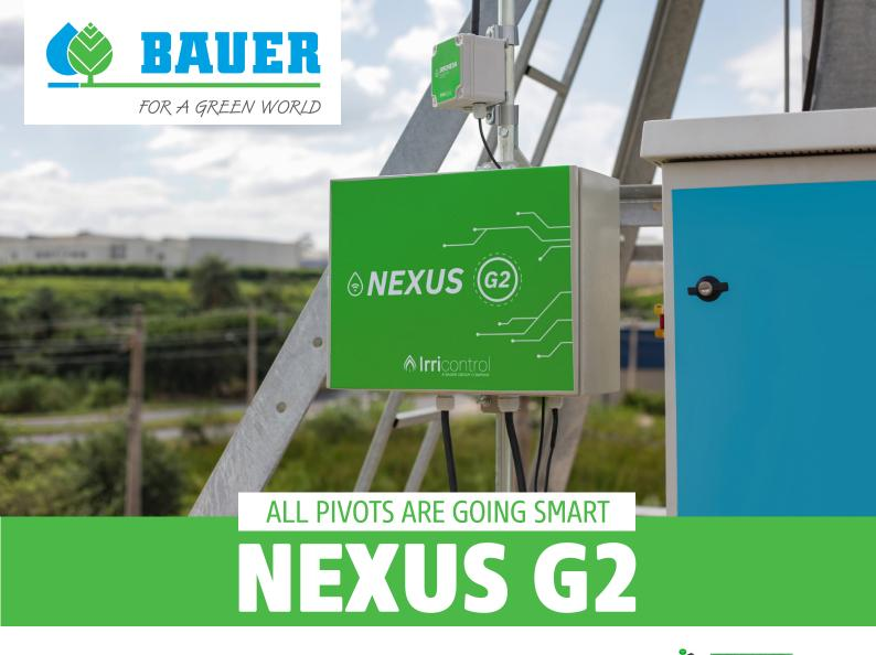
Installing a Nexus G2 offers opportunities to make the existing pivots smart, with their own radio infrastructure for reliable communication. This simplifies operation and makes it more efficient, with uniform control of all pivots via a single platform. The Nexus G2 control unit can be integrated seamlessly into control units of all pivot brands without any need to remove the old cabinet.
